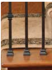
Open Tread Bottom Connection
