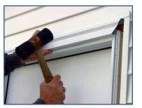
4. Screw jamb covers to the jambs. 5. Snap on the new brickmould.
