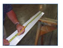
2. Measure door jamb & transfer dimensions to cladding.
